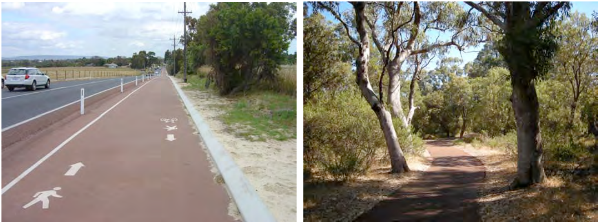
Above left: The pathway constructed along the busy West Swan Road in the Swan Valley is an excellent model for what could be achieved along Peppermint Beach Road and Stirling Road, to create a pathway link between Peppermint Grove Beach and Capel. Above right: The Tuart Walk, between Dalyellup and Usher, also provides an example of what the proposed pathway through the tuart forest on The Avenue road reserve might look like when constructed.
