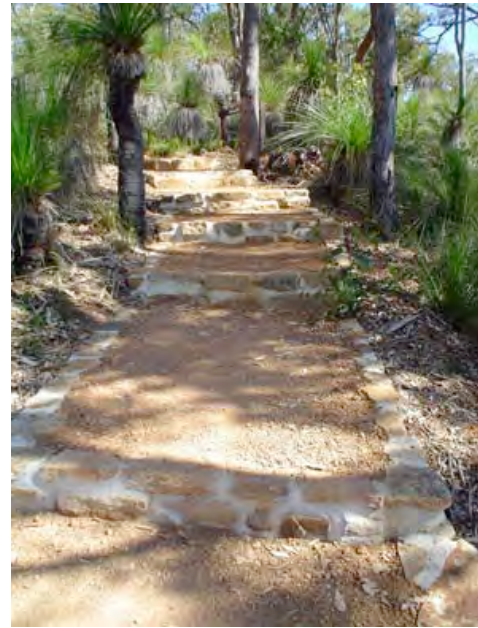
Quality construction, such as these rock steps on the Golden View Trail in Kalamunda, is the hallmark of a quality trail.
