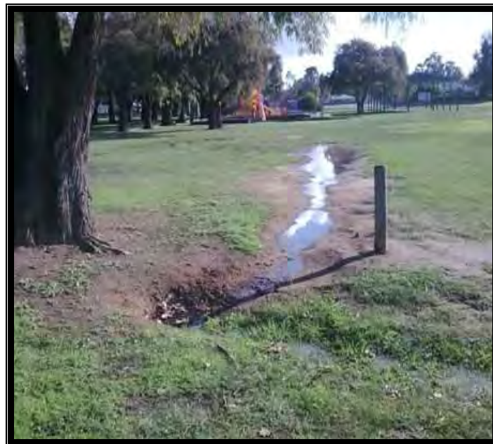
Inundation Photo B (Source: WGE, 2011)
