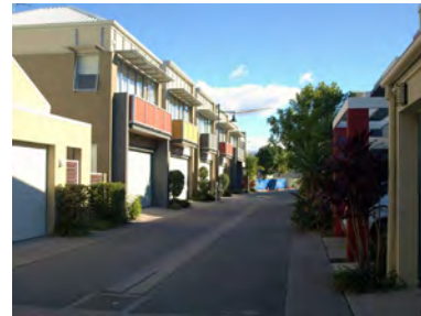
Rear laneways with building design creating opportunity for passive surveillance
