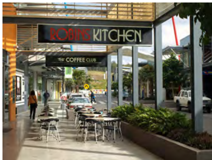
Shade structures protecting the pedestrian environment and encouraging public interaction
