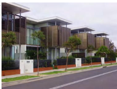
Use of low open fencing to define but encourage interaction with public/private realms
