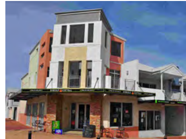
Ground floor commercial use with residential above
