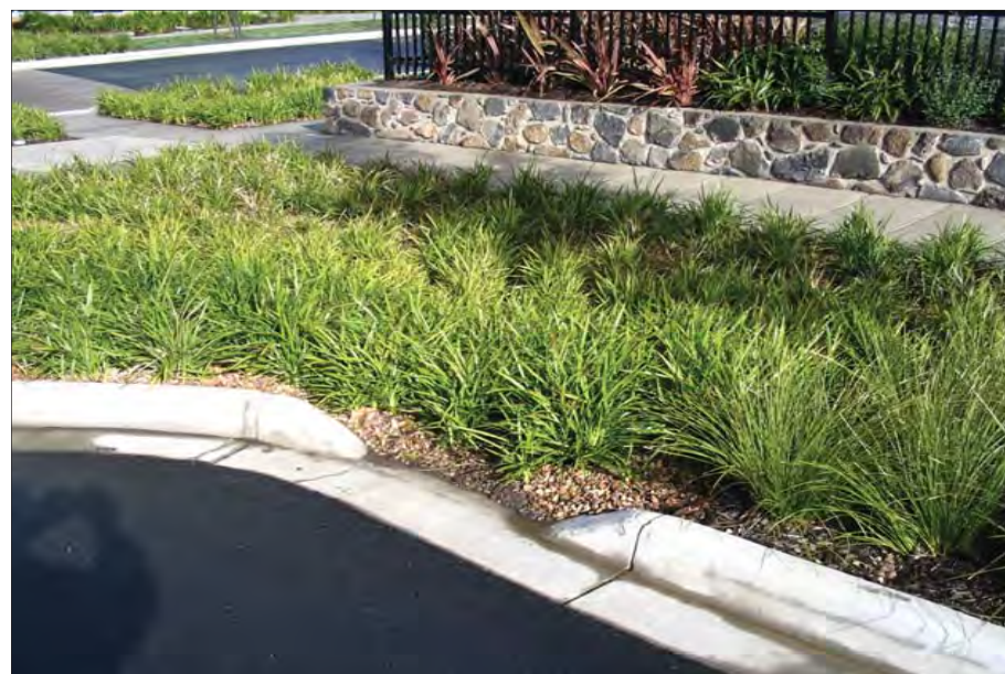
End of street bioretention unit
