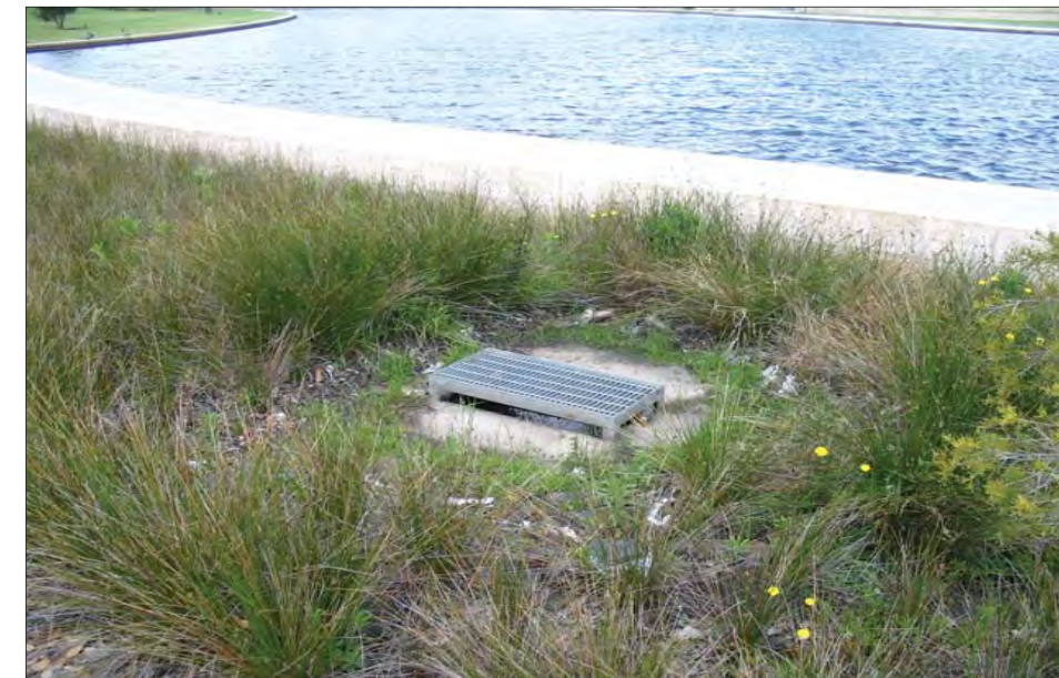
Bubble up pit in Bioretention Unit
