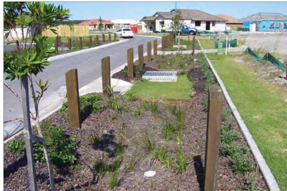
Streetside bioretention garden that filter water prior to infiltration to the groundwater
