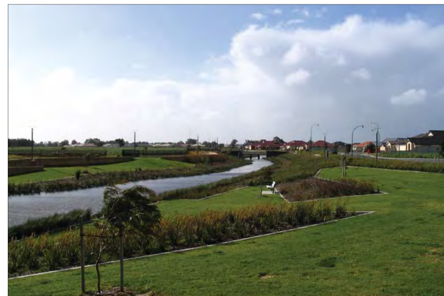
Bioretention swale in multiple use corridor that receives and transports groundwater as well as being an area of infiltration to groundwater.
