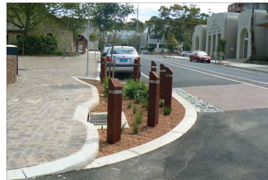
Streetside bioretention garden
