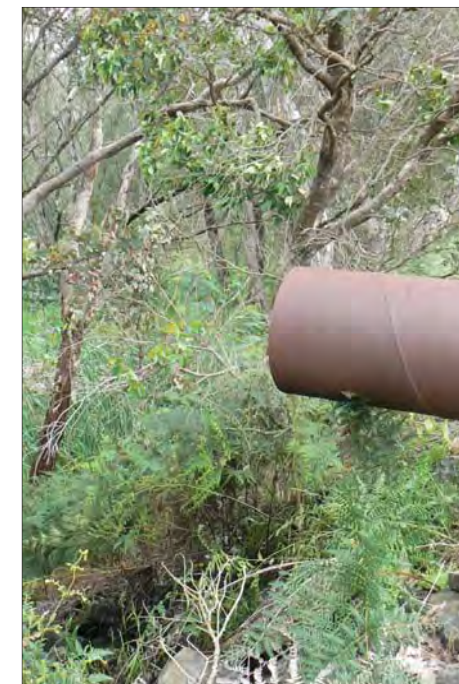
Discharge pipe from the dam into the Capel River gully
