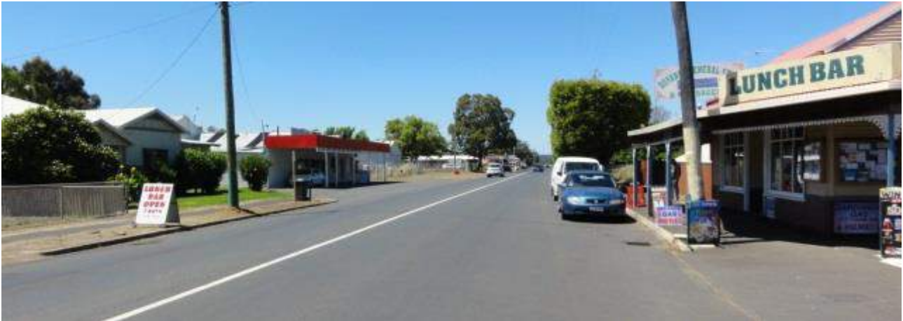
Figure 3-22 South Western Highway
