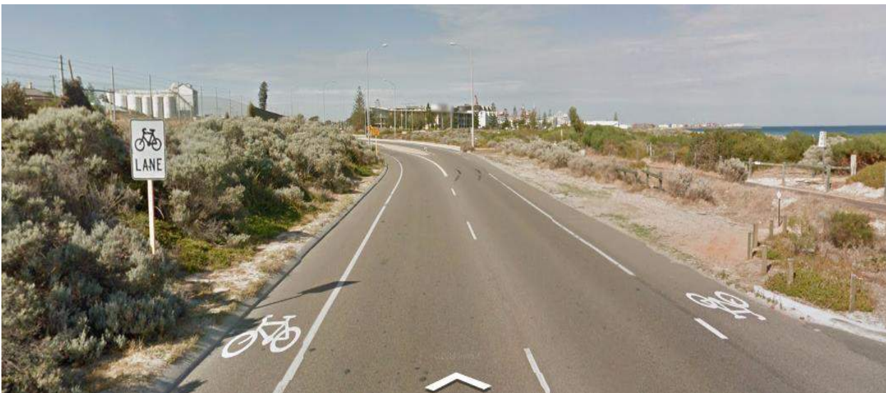
Figure 2-4 Standard Cycle Lanes - Curtin Avenue, City of Fremantle WA
