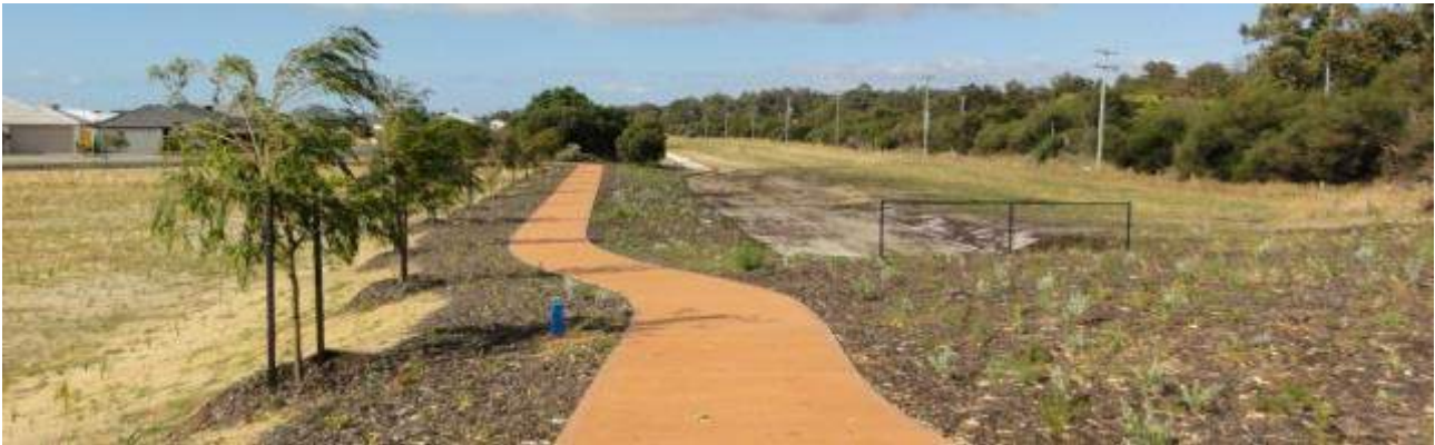
Figure 2-2 Shared Path – Shire of Capel WA
